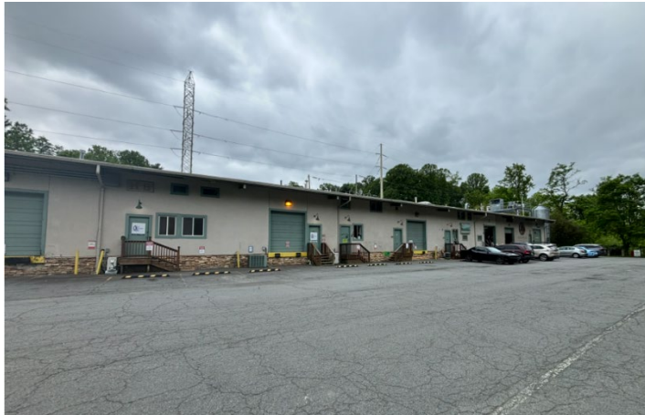
Figure 1 – Existing conditions photo of building from parking lot. Source: Staff photo.
