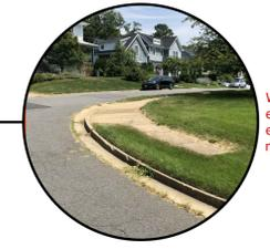
With this concept the sidewalk connects to the existing sidewalk along Holmes Dr NW. The existing ADA ramp would be replaced with a new (current standard) ADA ramp.
