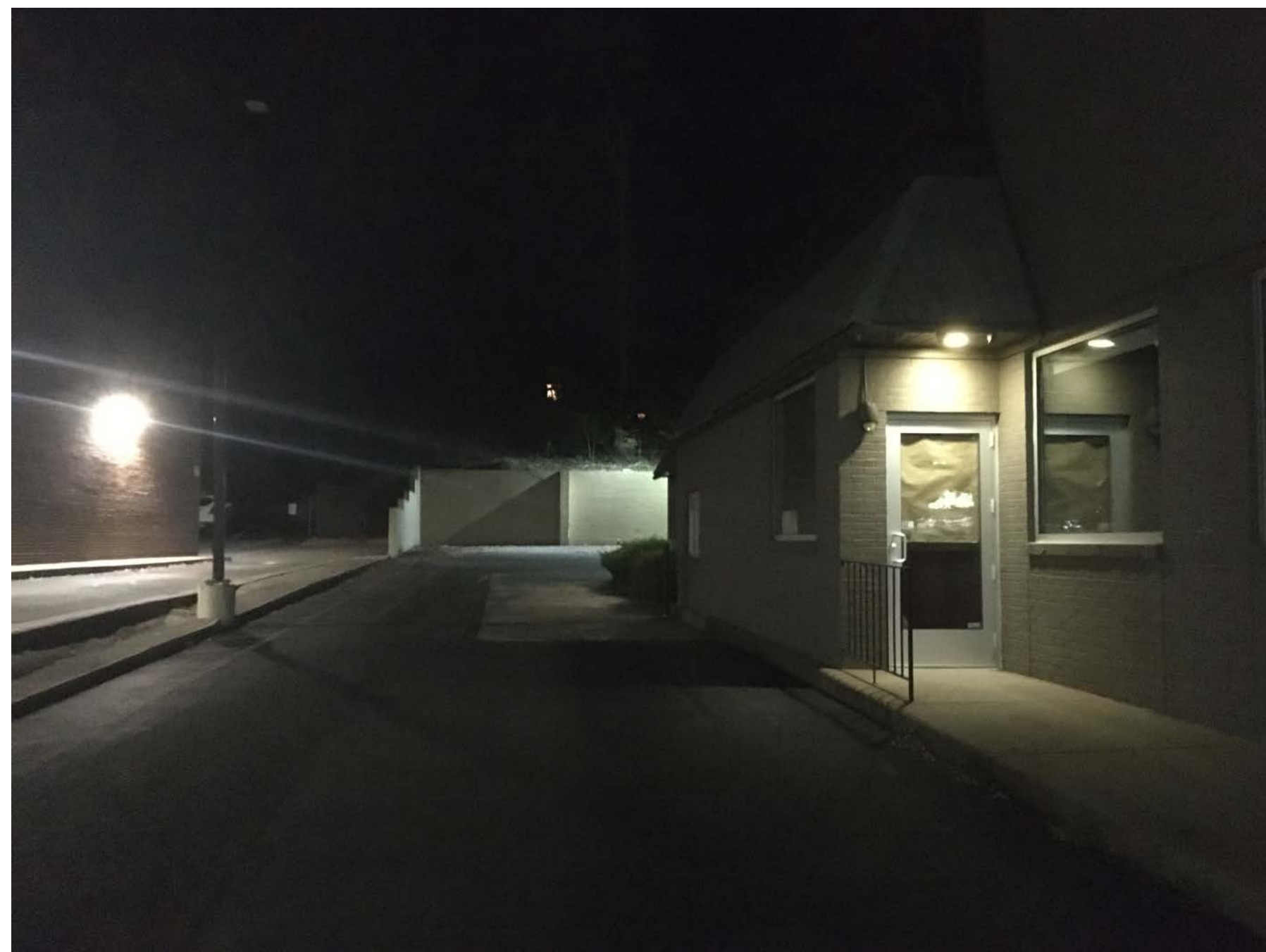
EXISTING POLE LIGHT AT LEFT SIDE OF BUILDING
