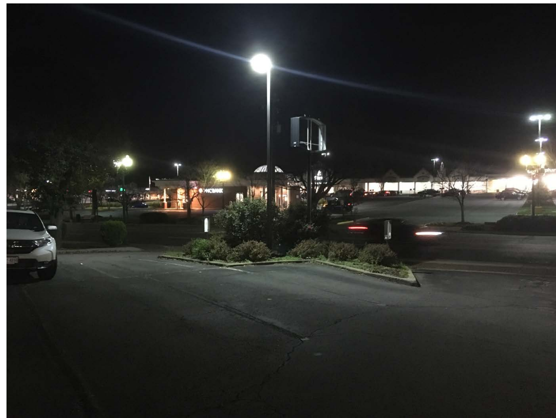
EXISTING FRONT POLE LIGHT
