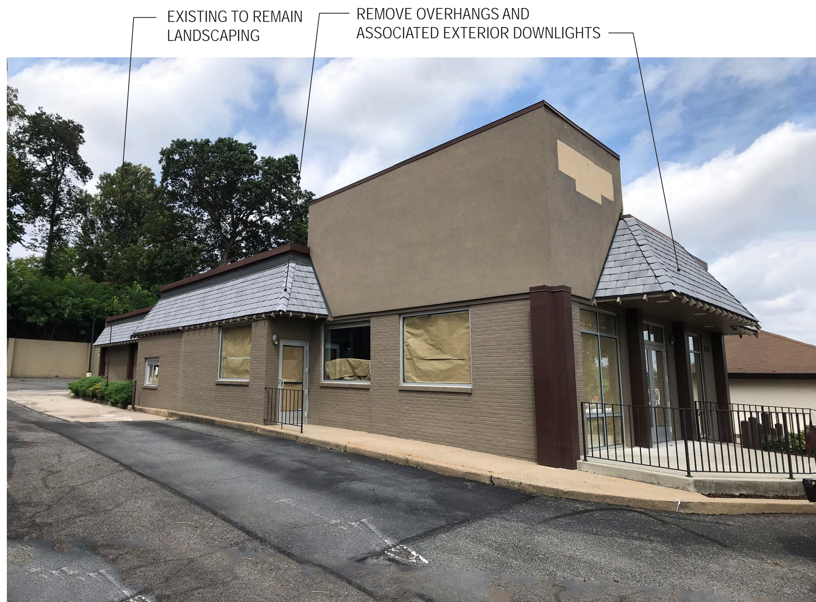
FRONT VIEW - EXISTING
