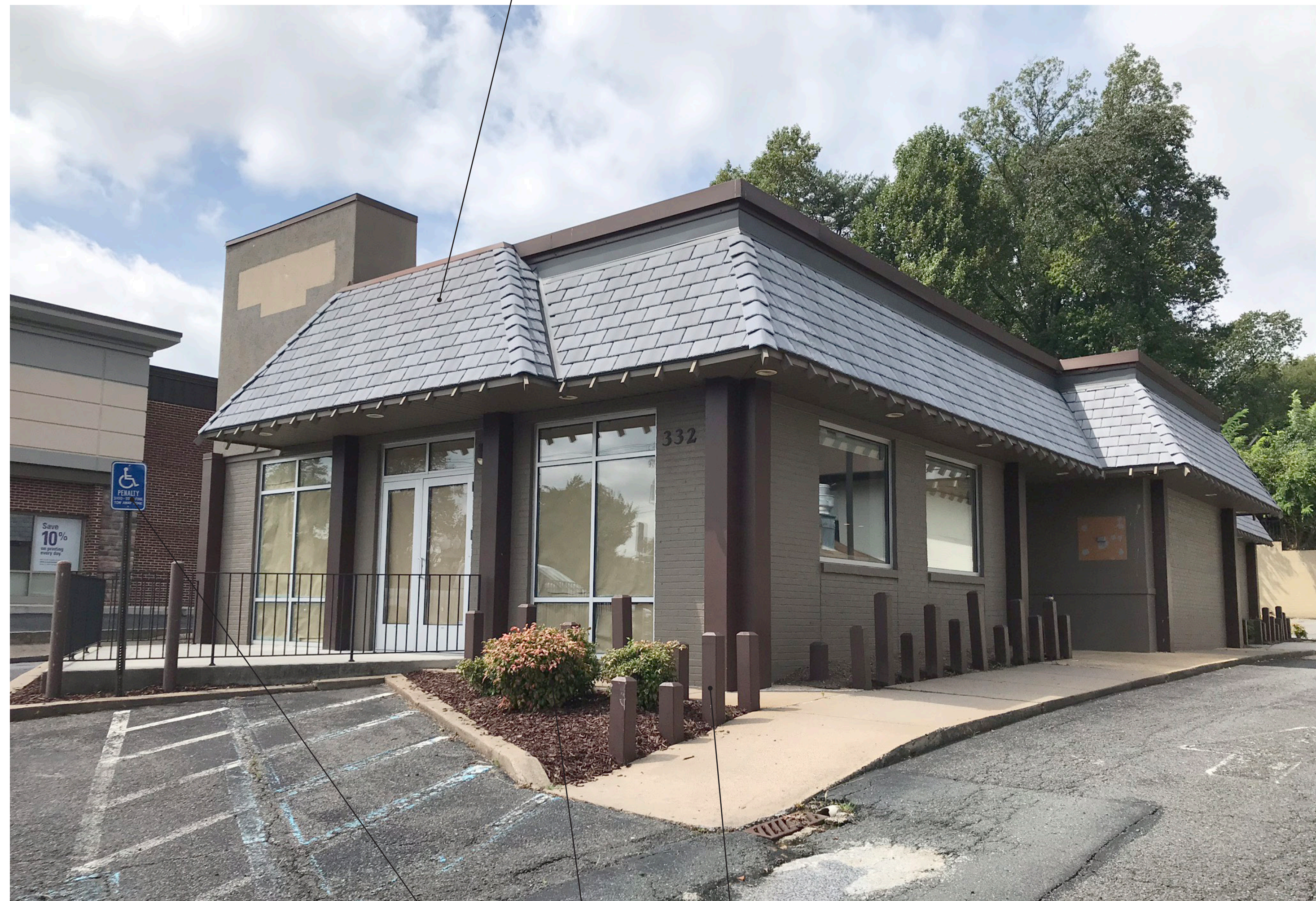
FRONT VIEW - EXISTING
