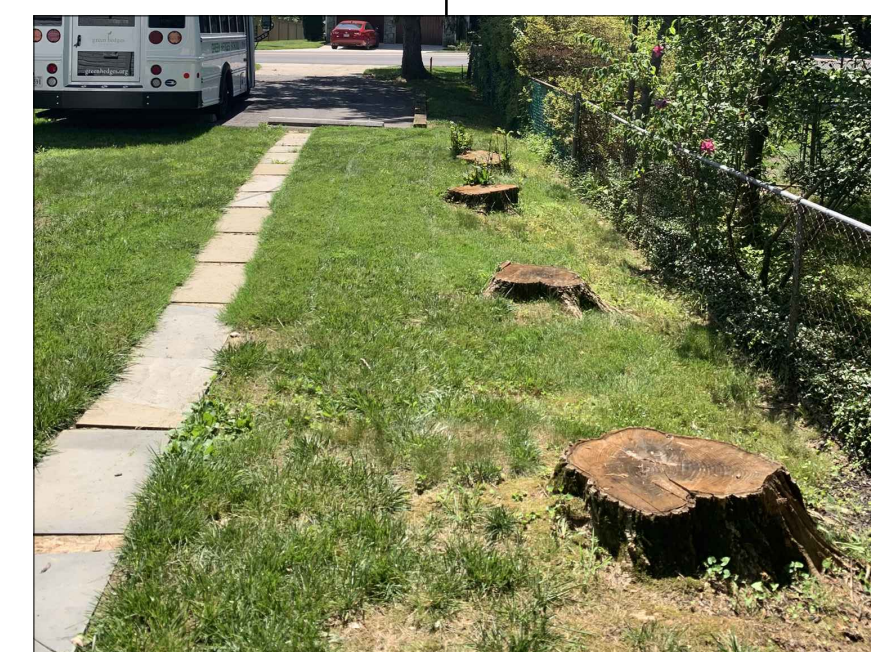
ON SITE VEGETATION HAS BEEN REMOVED
