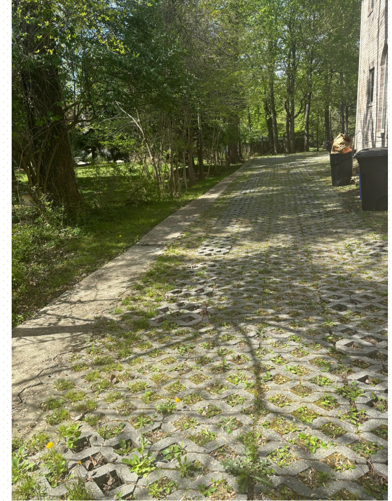
Continuation of driveway using grid pavers
