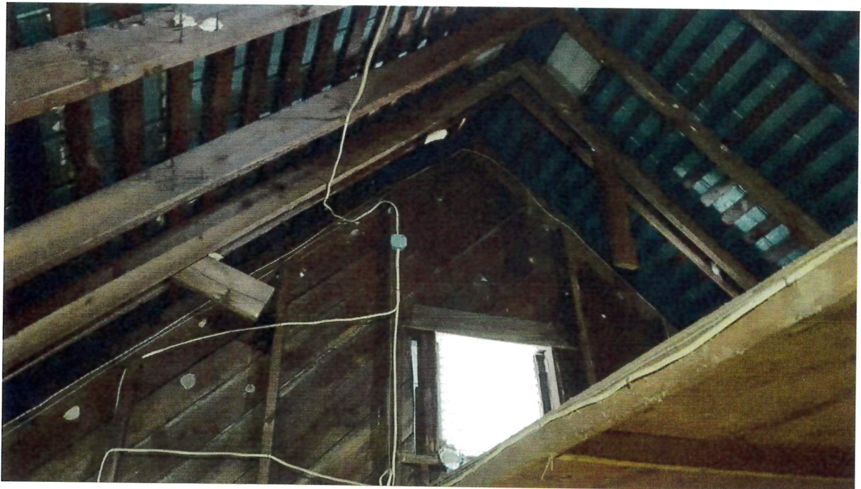
Photo #2 – View of Truss T2 showing several cut web members
