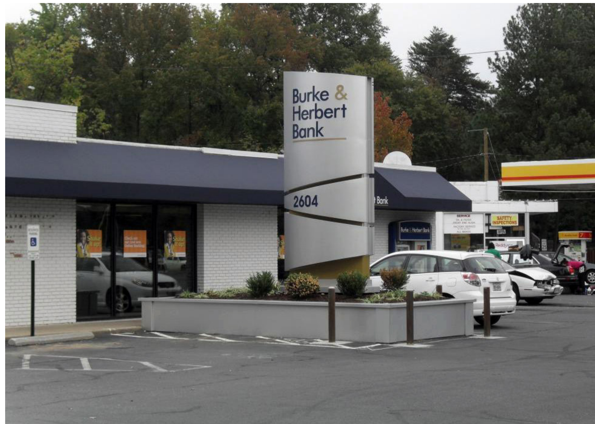
Existing Silver Pylon Sign Sherwood Hall Lane, Alexandria, VA
