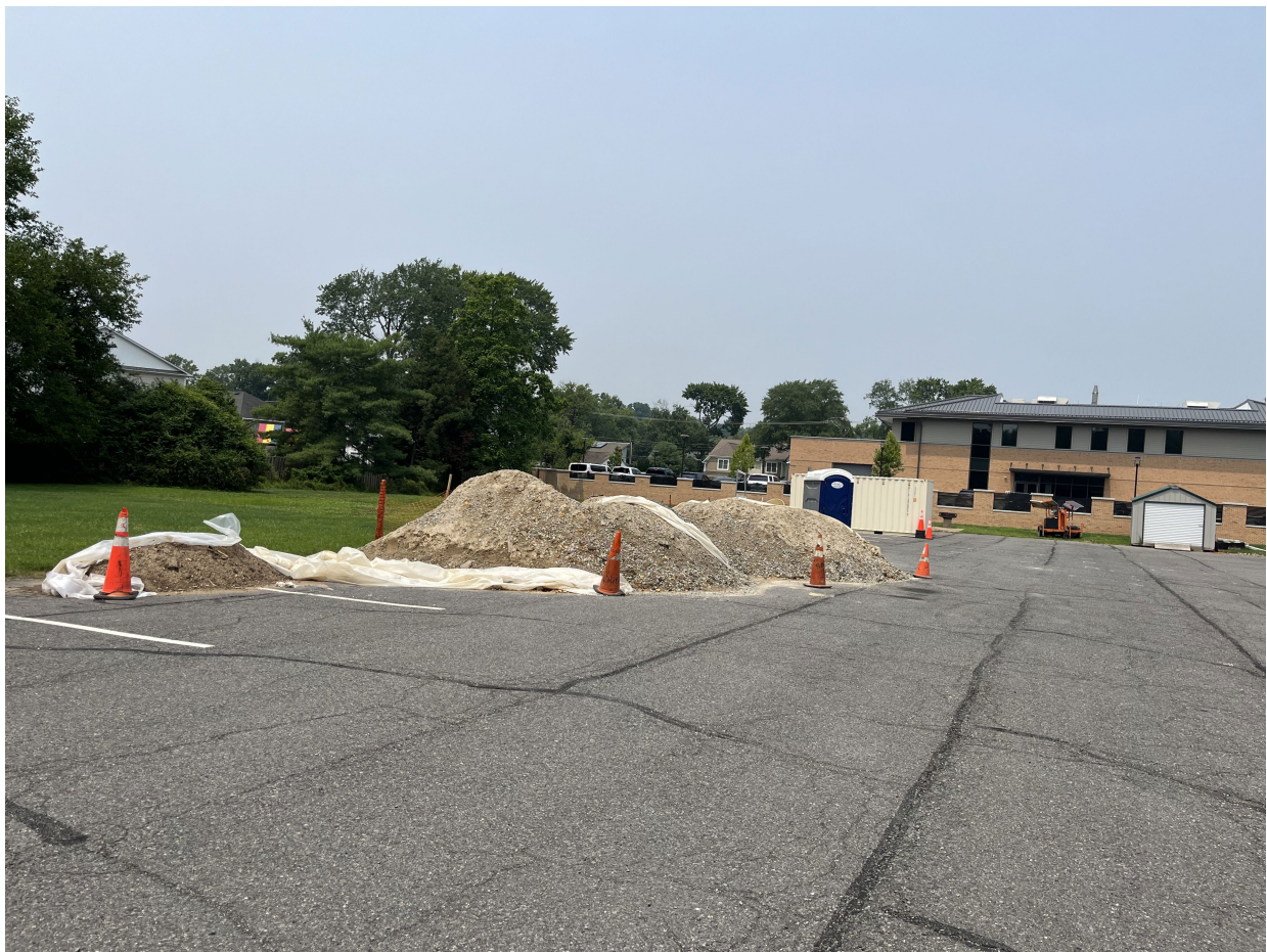
Photo 2: Previous stockpile of aggregate material used in a water main replacement project in 2023. Any stored aggregate material would be covered with a tarp to prevent any stormwater runoff pollution and no hazardous materials, spoils, or salt will be stored at 301 Center St S.
