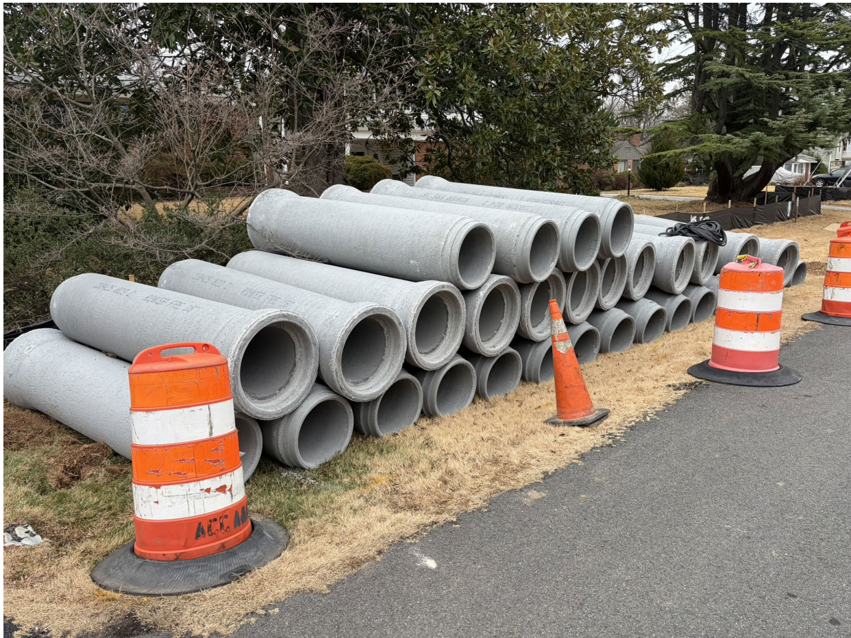
Photo 1: Staging of concrete storm drain piping at the Glen Ave sign. Given the proximity of 301 Center St S to properties with high traffic of children, orange safety fencing would be provided around any proposed stockpile or staging of equipment.
