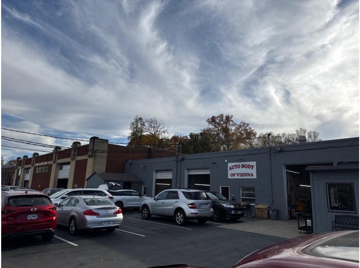
Existing property at 330 Dominion Rd. NE, left side.
