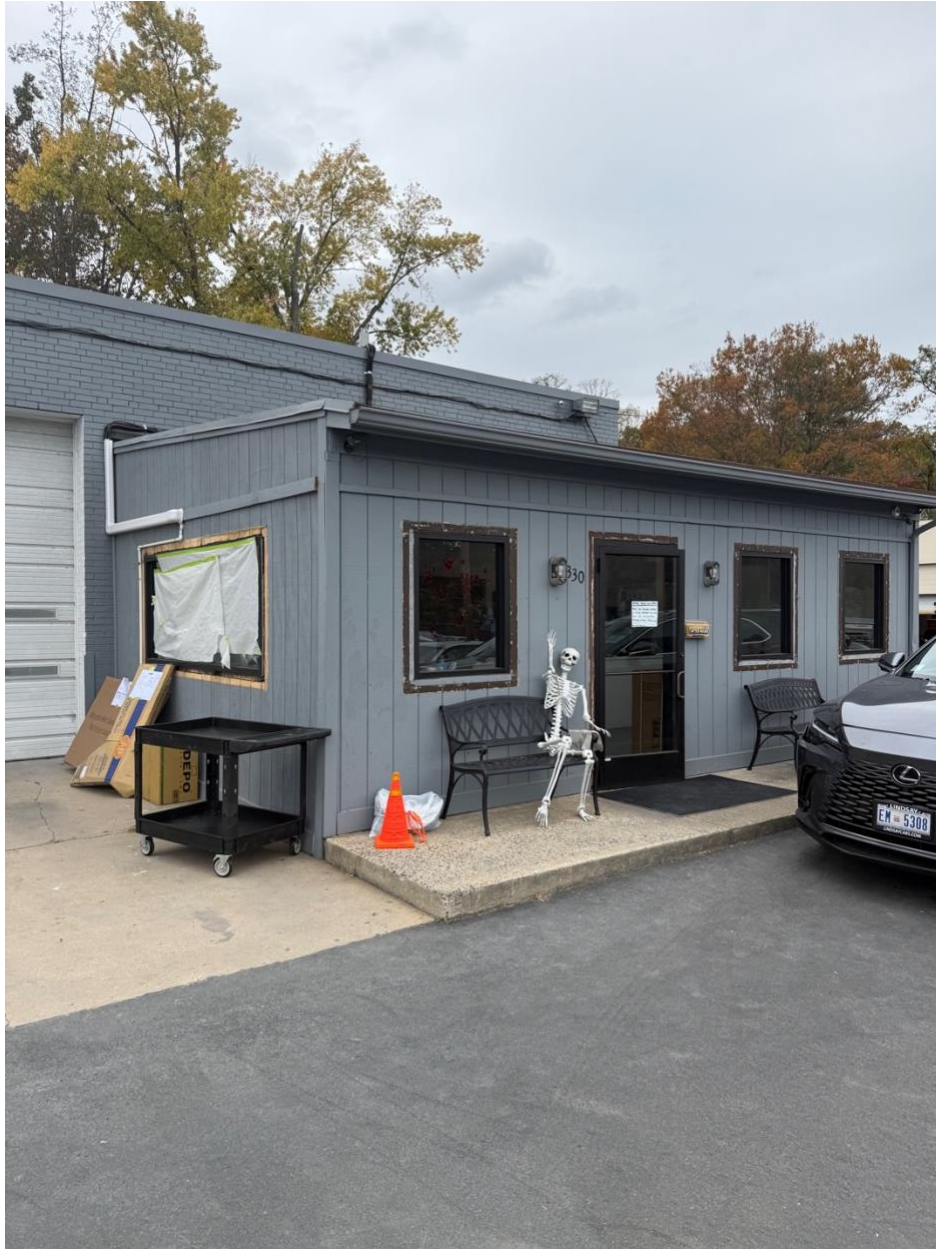
The existing structure to be wrapped, isolated.
