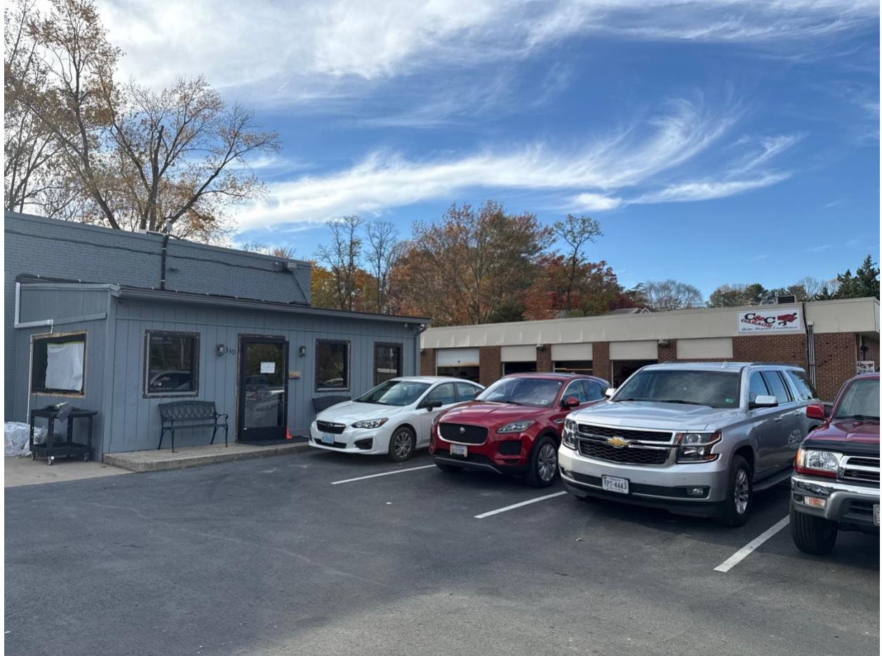
Existing property at 330 Dominion Rd. NE, right side.
