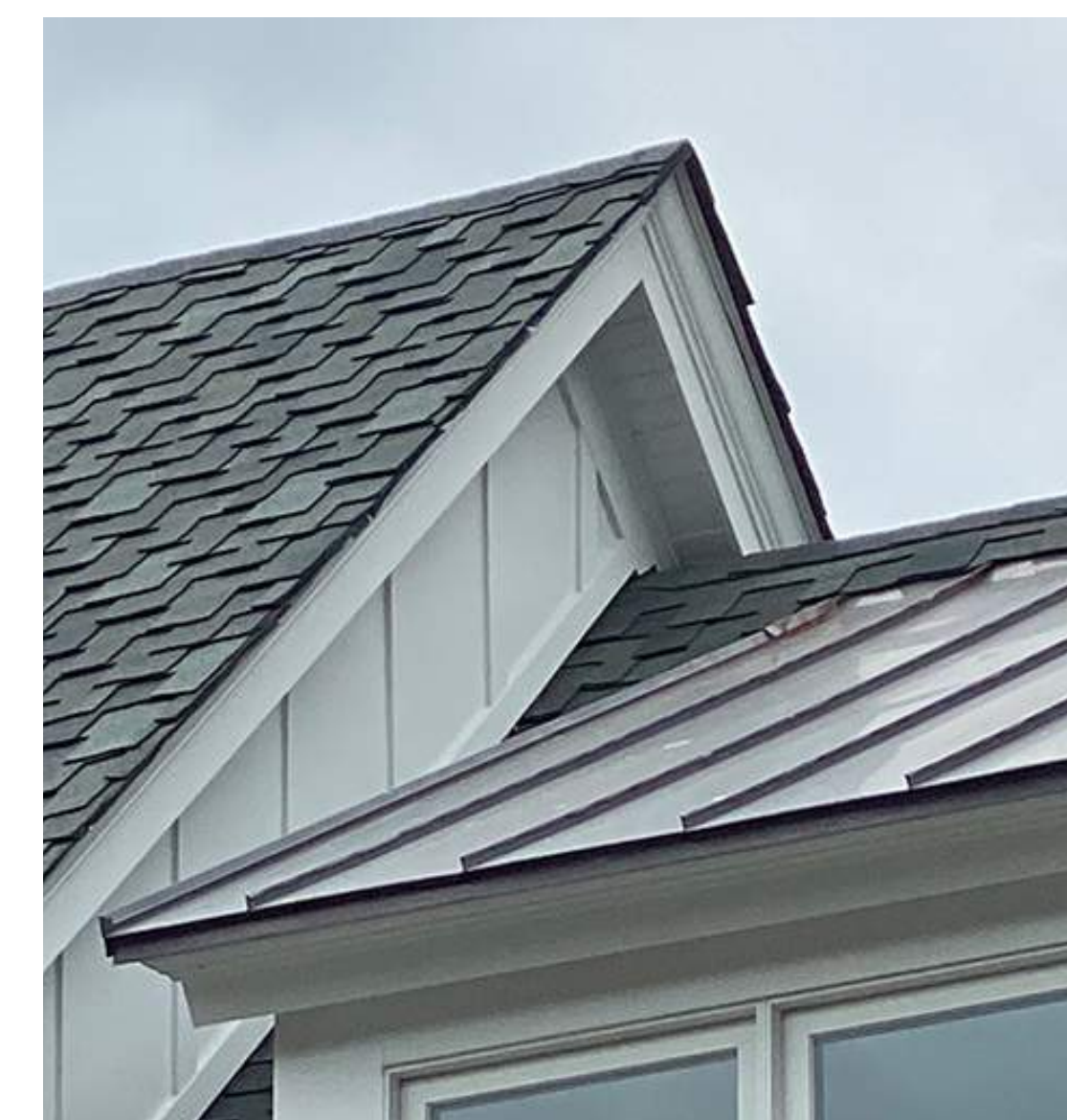
SLOPING COMBO ROOF: SHAKE AND METAL STANDING SEAM
