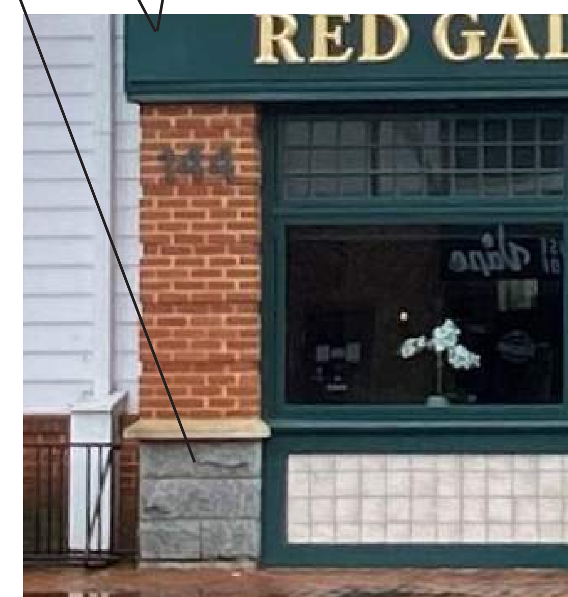
STONE BASE AT BRICK COLUMN & DECORATIVE MOLDING AROUND STOREFRONT
