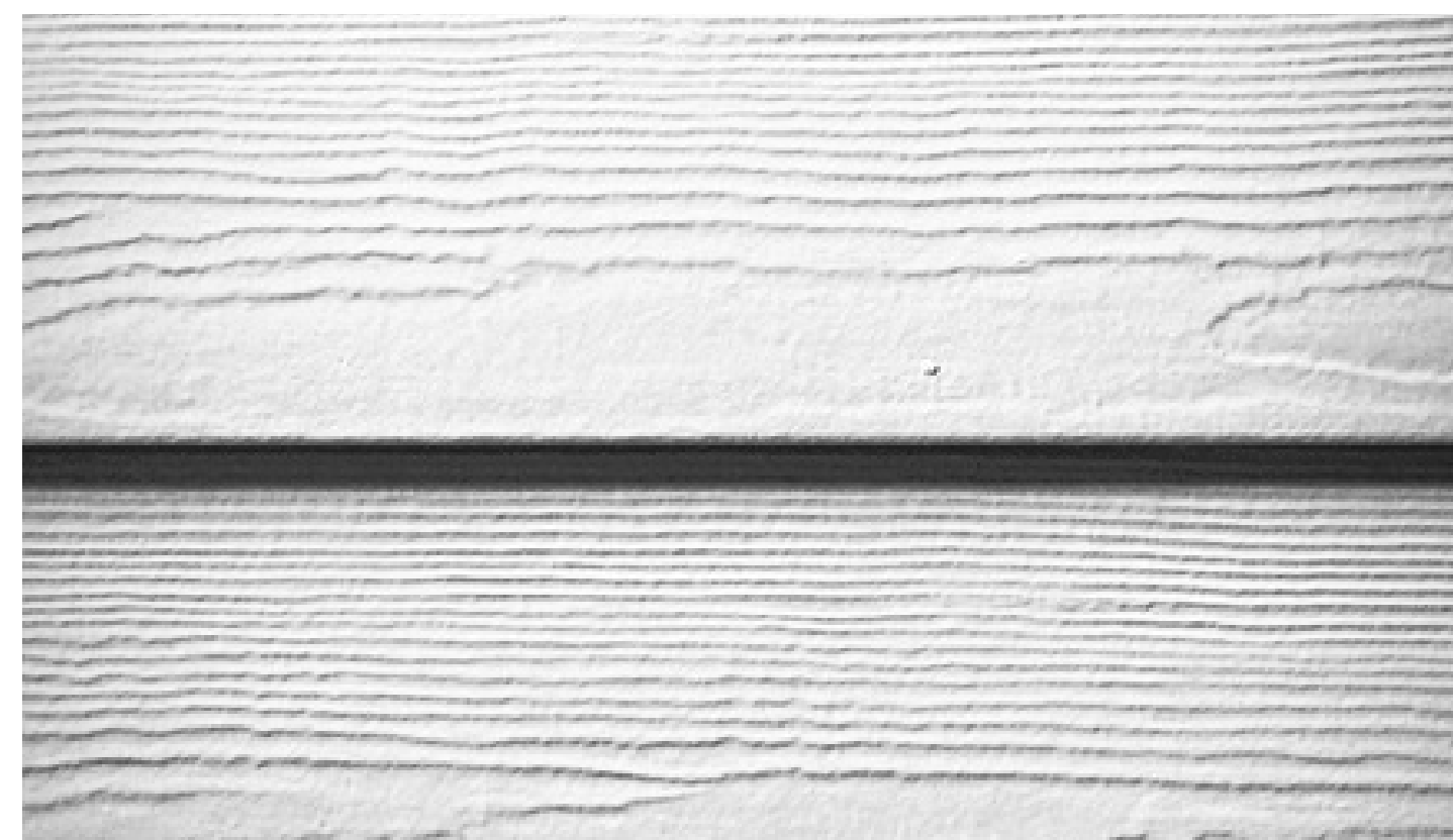
② CEMENT BOARD SIDING, MANF: JAMES HARDIE; PRODUCT: HARDIE SIDING COLOR: SW2831 CLASSICAL GOLD, SW LINK GRAY
