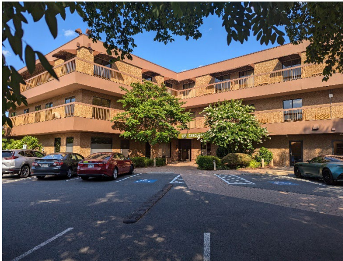
Figure 1 – Building entrance to 3 rd floor Suite 302 Source: Staff Photo
