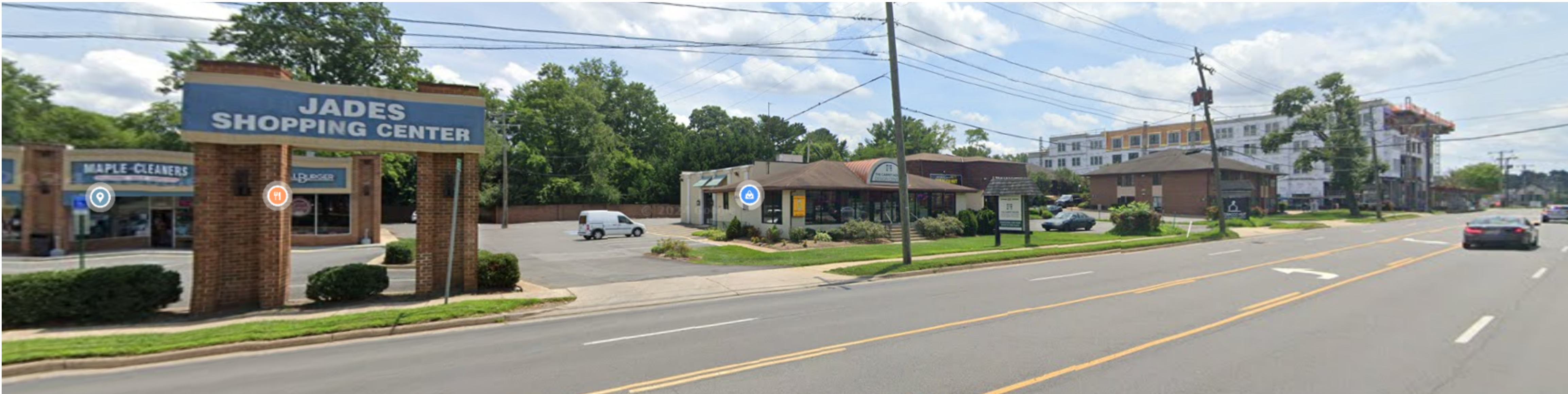
BUILDING ON RIGHT SIDE
