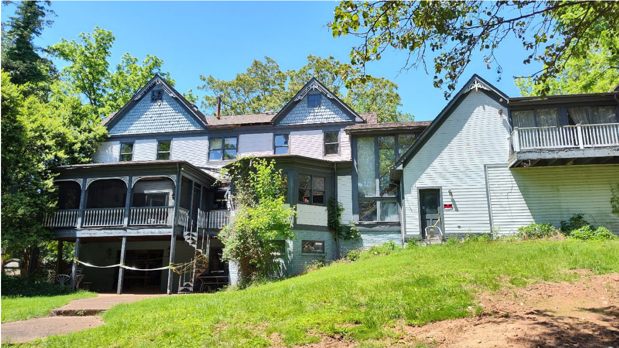
Photo of 288 Windover Ave – Rear
