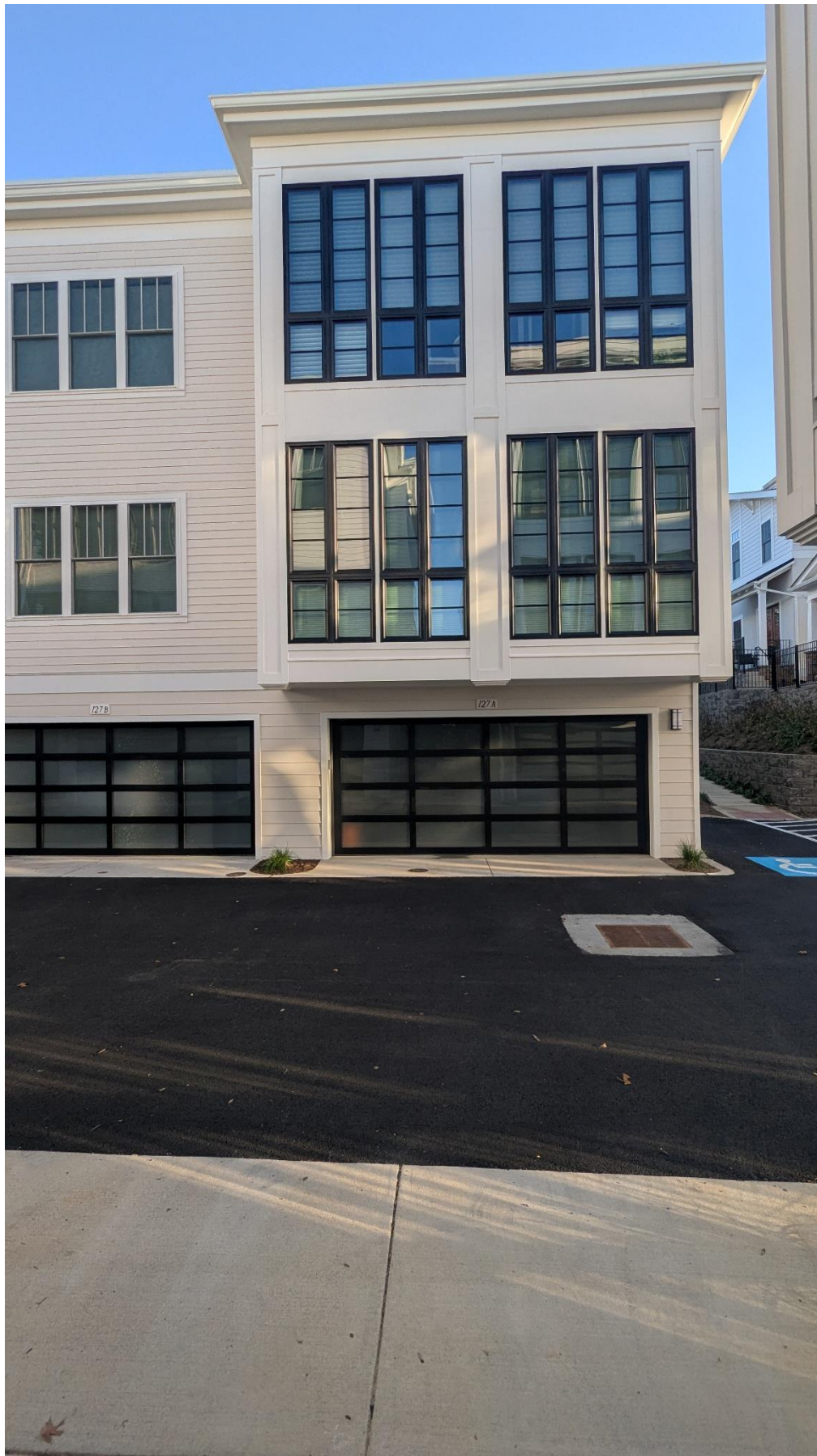
Rear view of 127A Park Street NE
