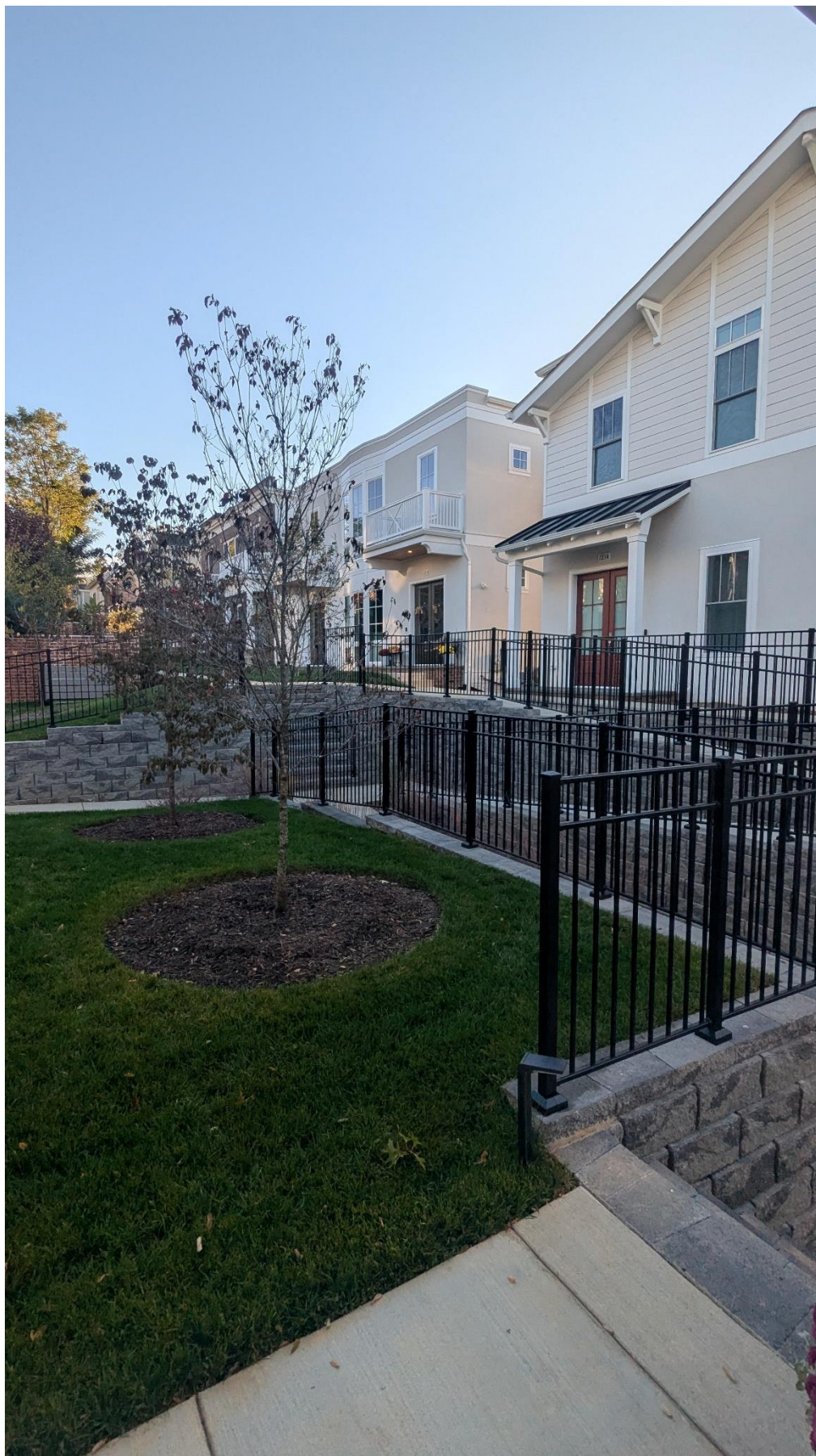
View from front 127A Park Street NE
