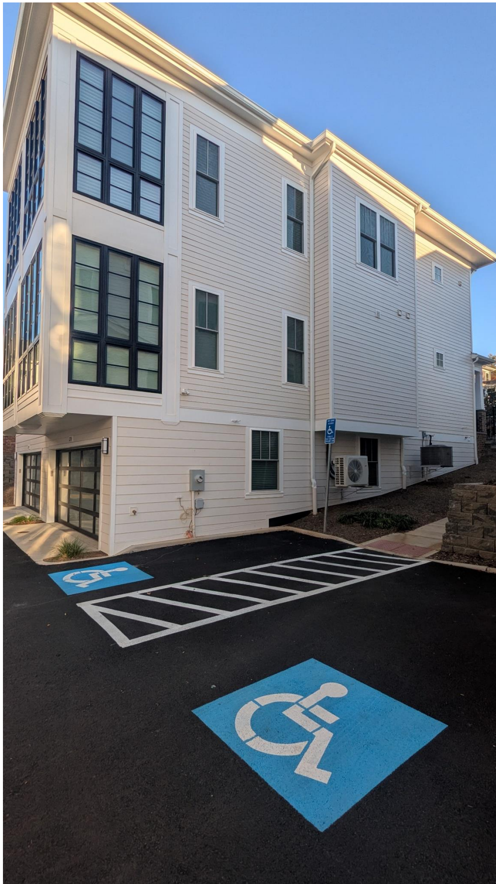
Additional side view of 127A Park Street NE Note: Conduit from roof is run internally to the electrical panel
