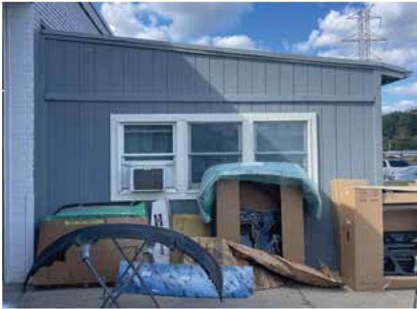
Wrapping white window frames
