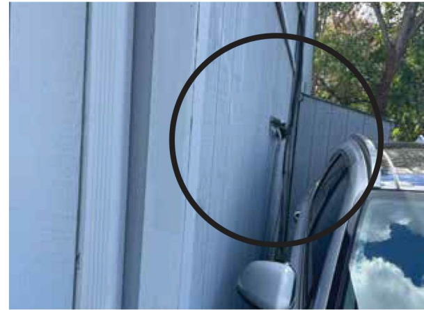
Wiring. Wrap underneath
