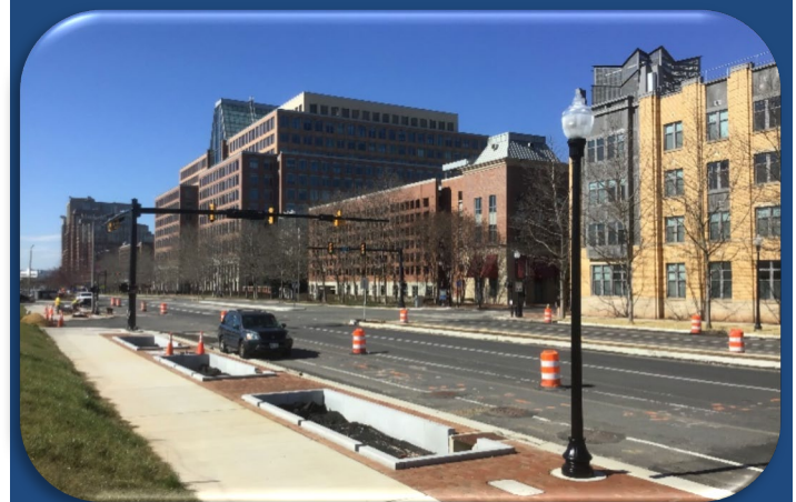
Eisenhower Avenue Roadway Widening Project, Before (top), Construction (middle), CA/CI (bottom)
