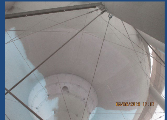
Recoating of the Third Street Tank
