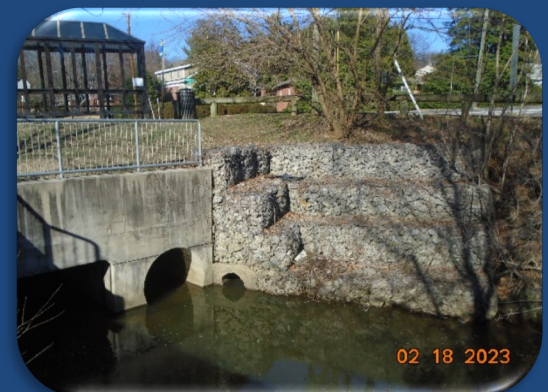
WRA assesses stream morphology as part of the semi-annual bridge inspections in Vienna.US Merchant Marine Academy – Mallory Pier
