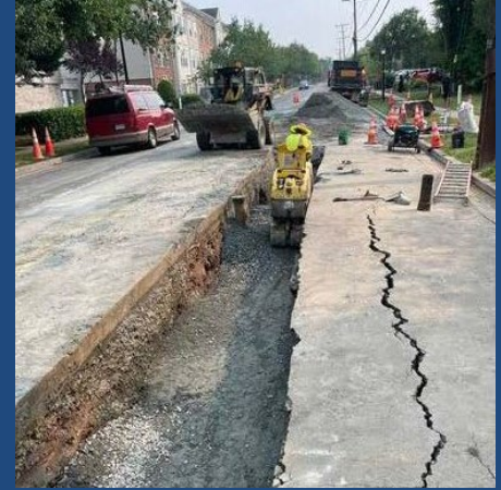
Center Street Water Main Replacement, Town of Herndon
