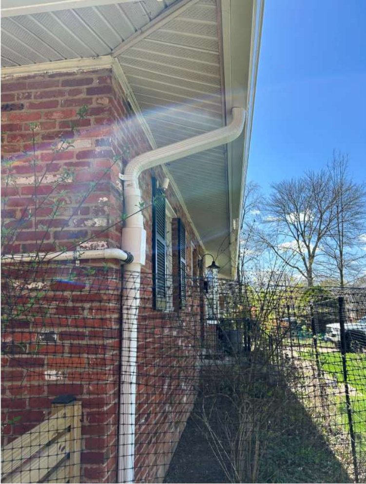
Pipe from front downspout to cistern
