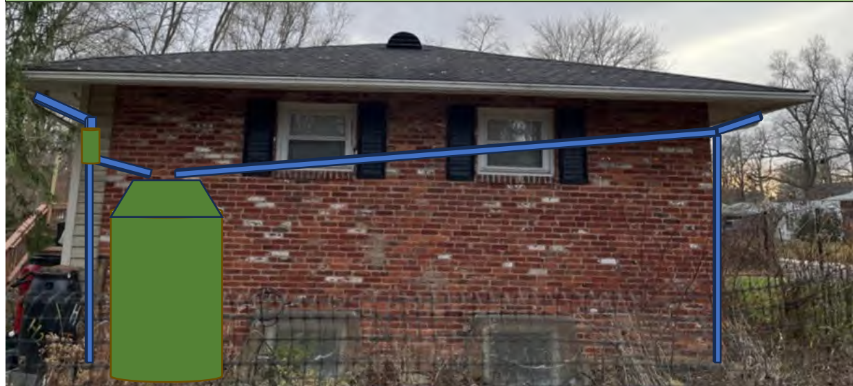
Project Site (After)
