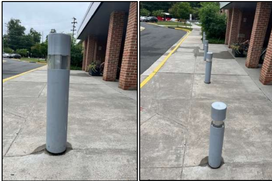
VCC Building Bollards
