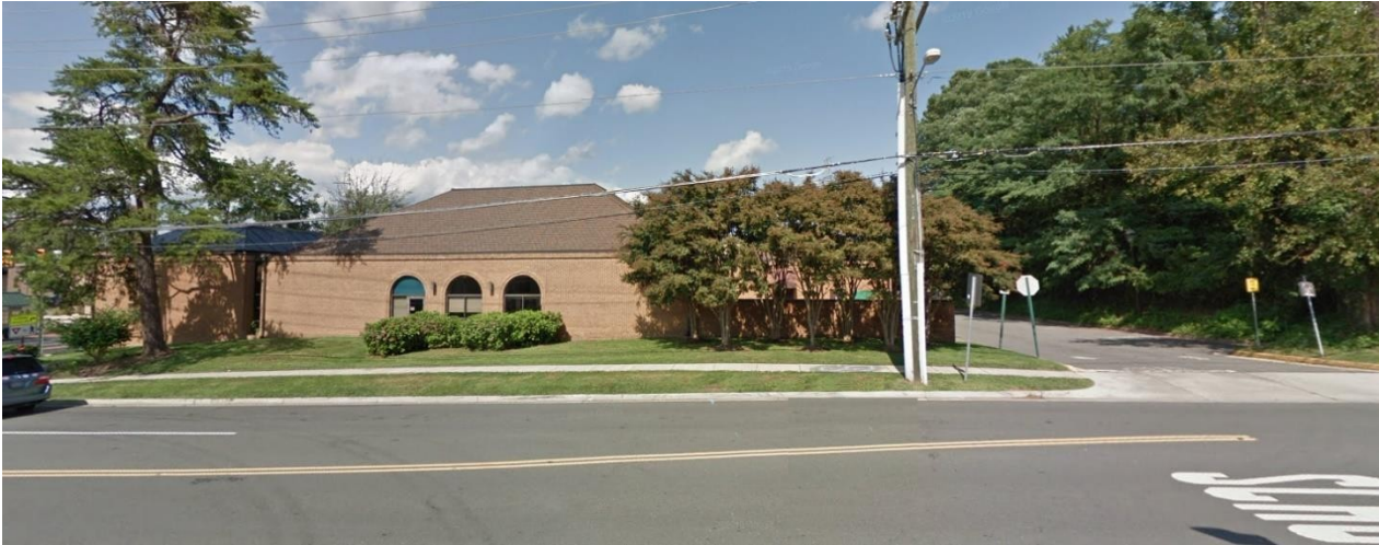
Existing Library – Center Street façade
