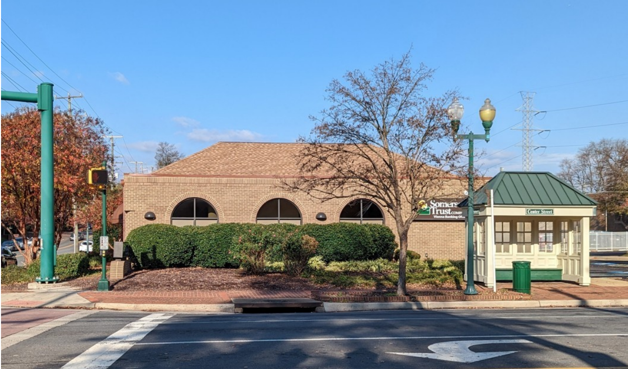
Adjacent property opposite on Maple Avenue: Somerset Trust Company
