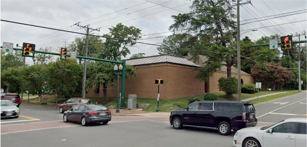
Existing Library from the intersection of Maple Avenue and Center Street
