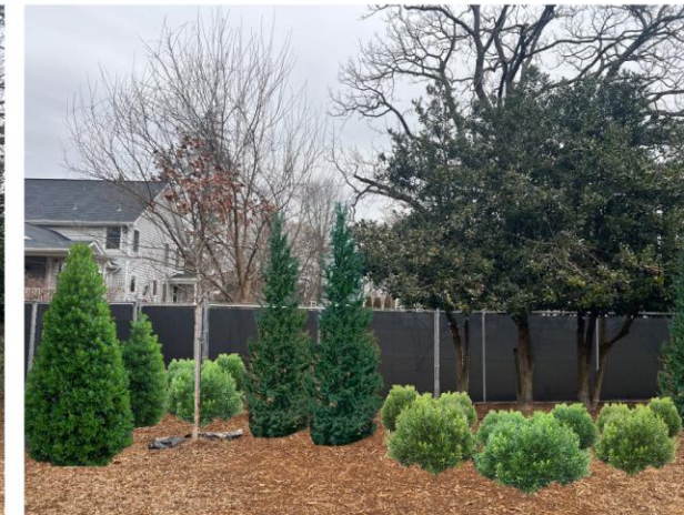
Existing chainlink fence with Acoustiblok panel & planting buffer
