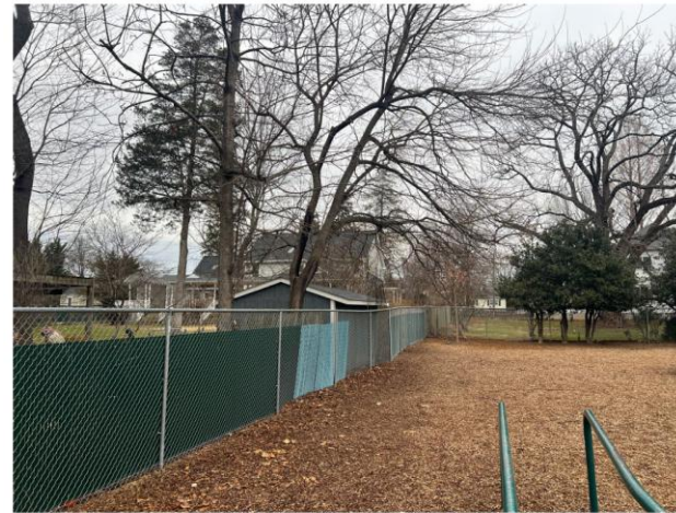
Existing chainlink fence
