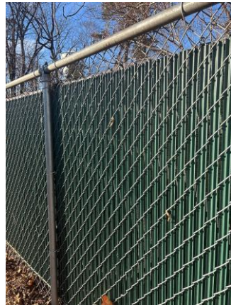
Existing chain link fence
