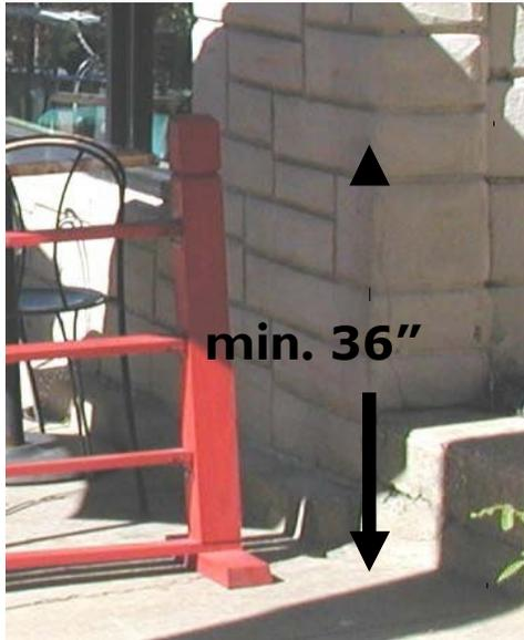
*Sectional fencing barrier height must be at least 36\"/>*
