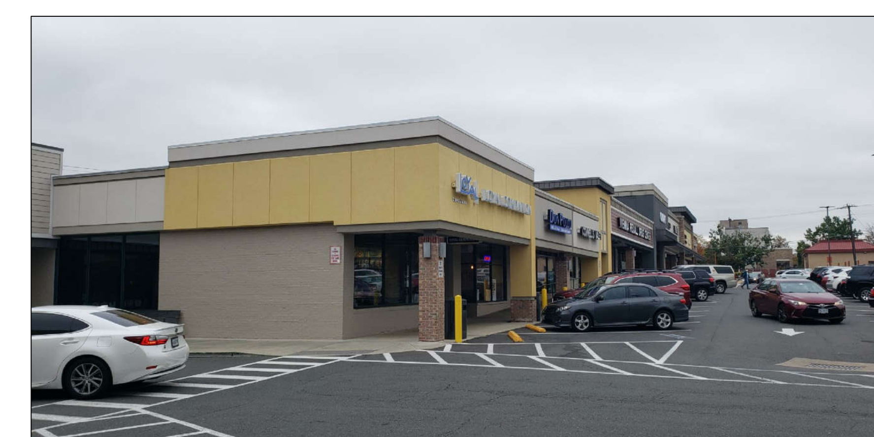
B PHOTO - EXISTING ADJACENT BLDG scale: NTS
