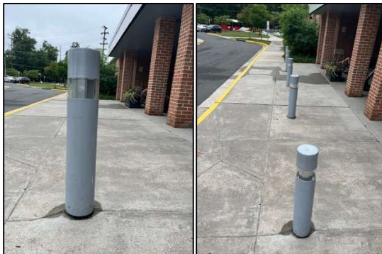
VCC Building Bollards
