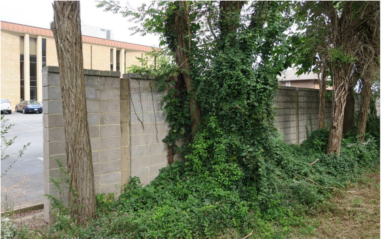
Figure 2 - Existing masonry wall along Glen Avenue Southwest
