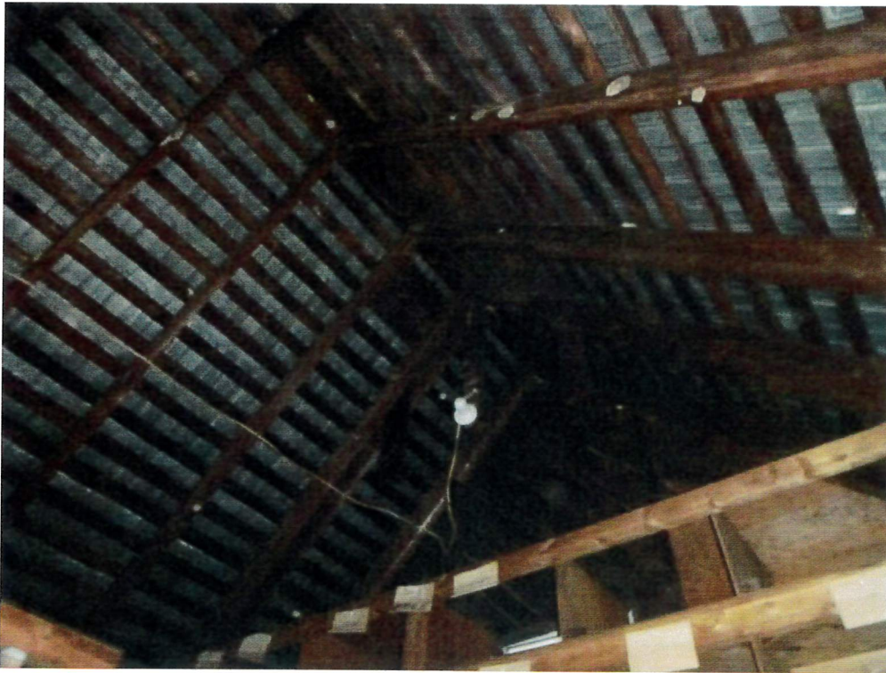
Photo #6 – Typical existing roof construction – rafters only, all web members removed
