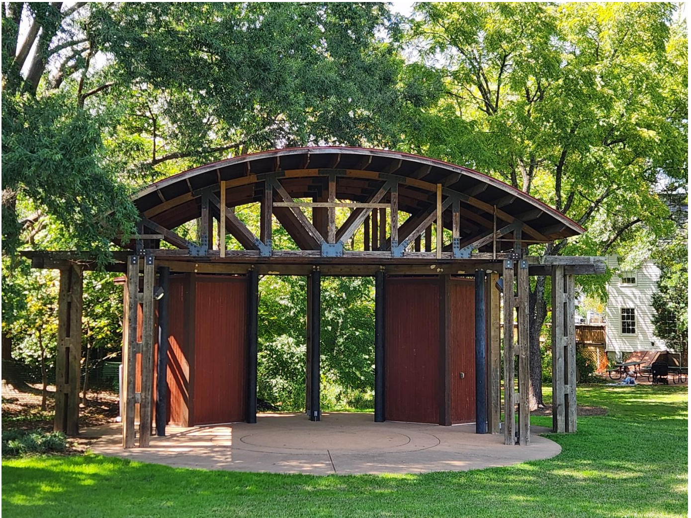
Figure 2 – Overall elevation view of amphitheater
