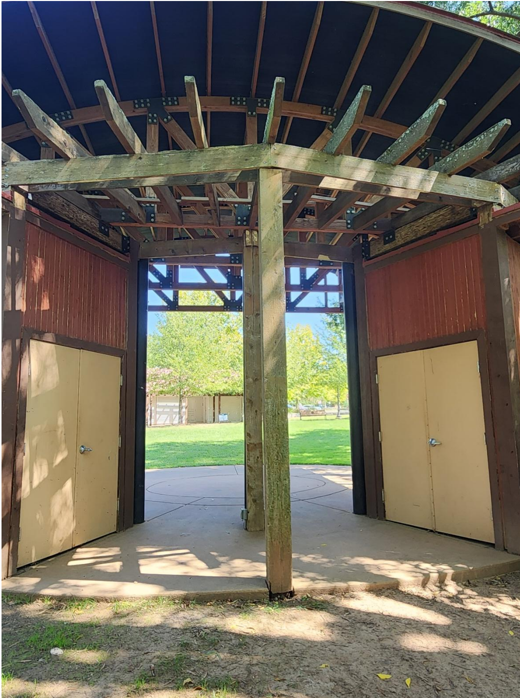
Figure 5 – Open trellis and storage sheds at rear of amphitheater
