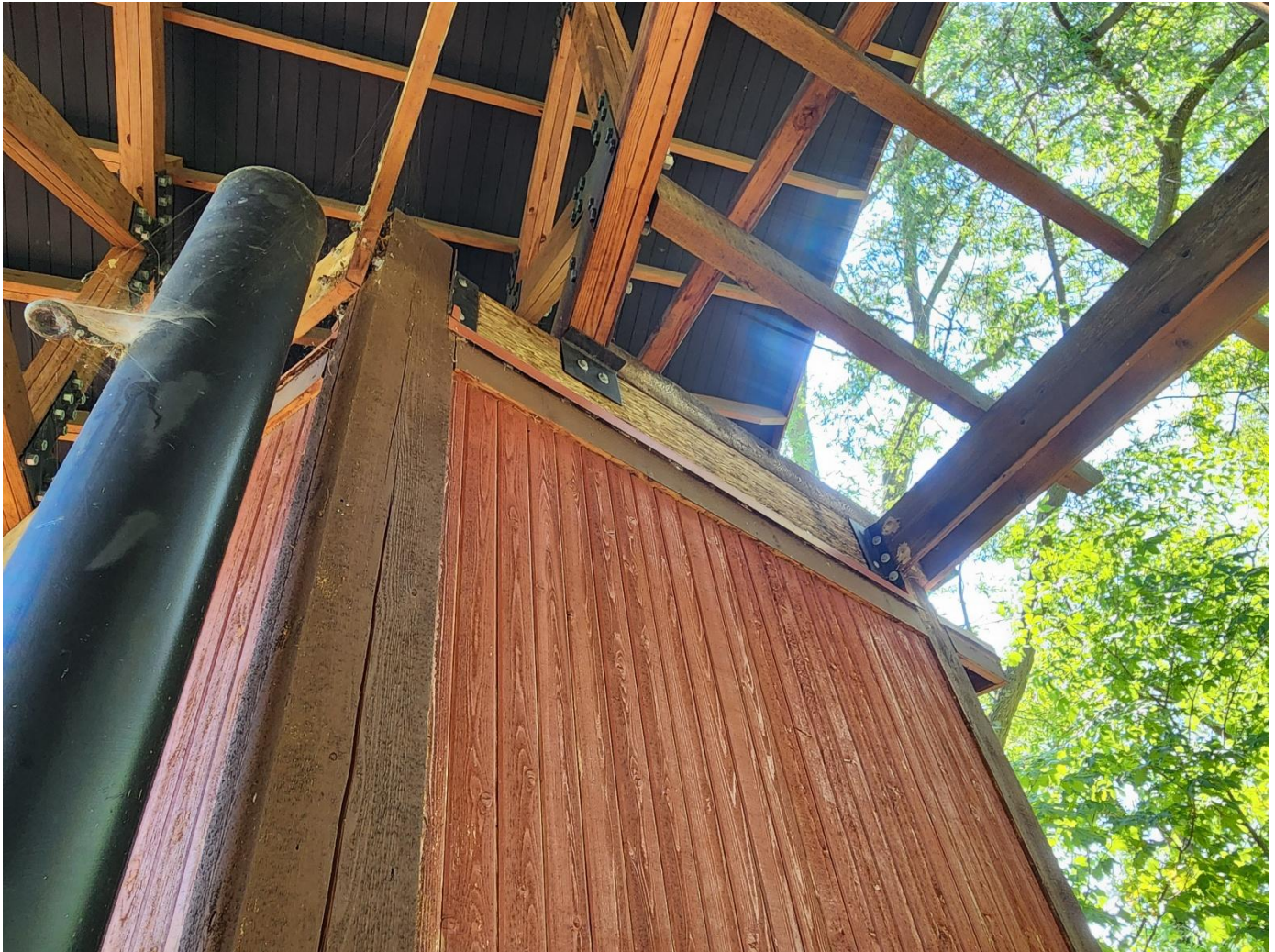
Figure 7 – Top of existing storage shed area
