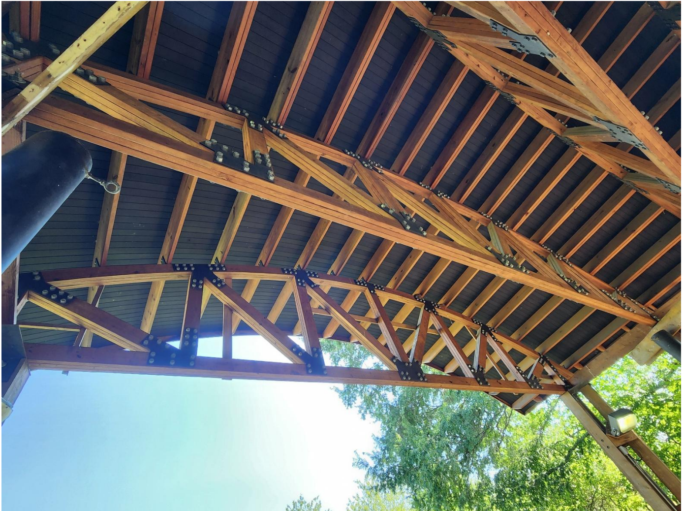
Figure 6 – Underside of barrel-vaulted roof showing wood trusses
