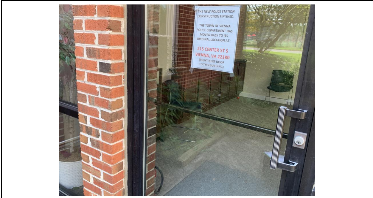
Homogeneous Material No. 32 – ACM White exterior door caulk located on the front entrance door and exterior door on left side of building.
