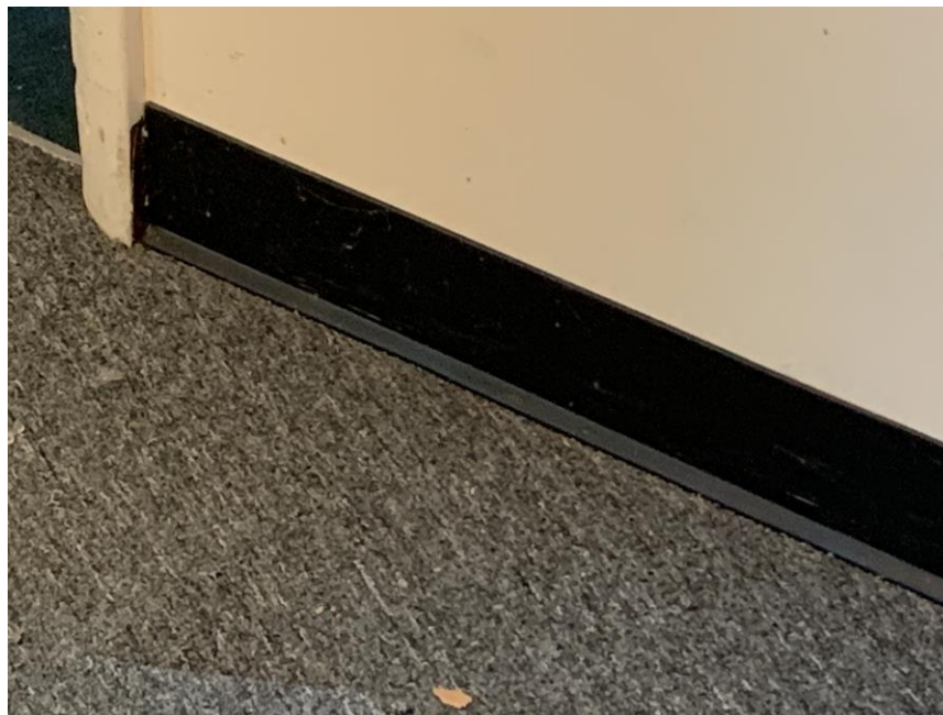
Homogeneous Material No. 8 – Non-ACM 4" Brown Vinyl Cove Base with associated tan mastic located in Rooms 1 and 2 adjoining the Sanctuary.
