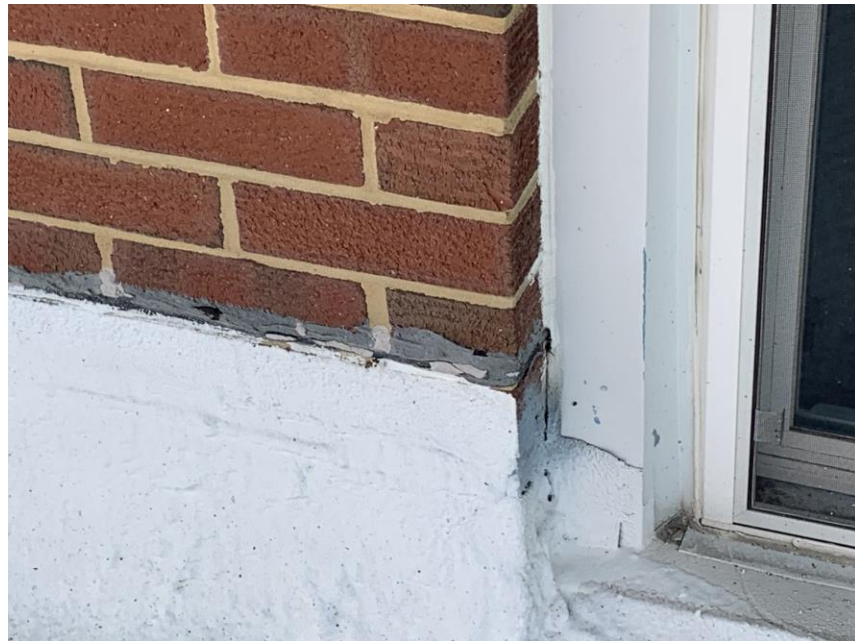
Homogeneous Material No. 2 – Non-ACM Black Roof Flashing Caulk located on building roof (flat part).
