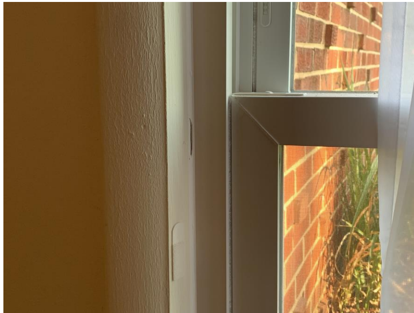
Homogeneous Material No. 10 – Non-ACM White Interior Window caulk located in Rooms 1 and 2 adjoining Sanctuary.
