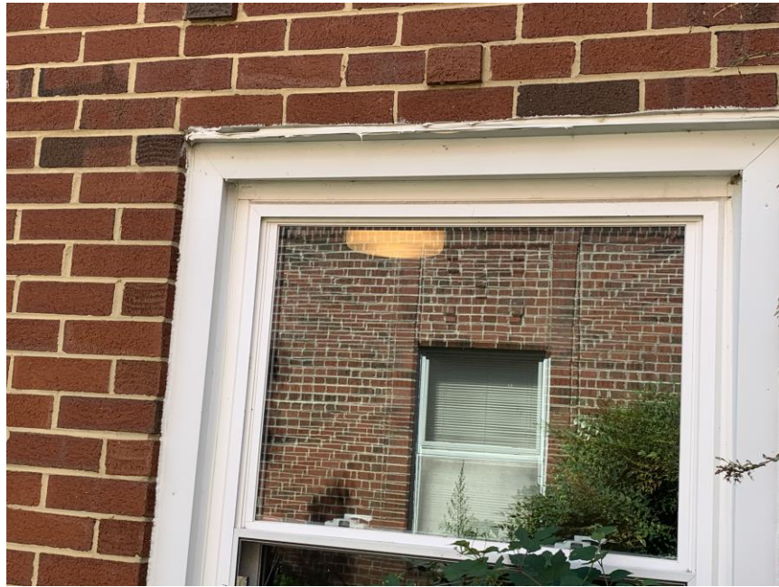
Homogeneous Material No. 33 – Non-ACM White exterior window caulk located on the Left and right-side exterior windows.
