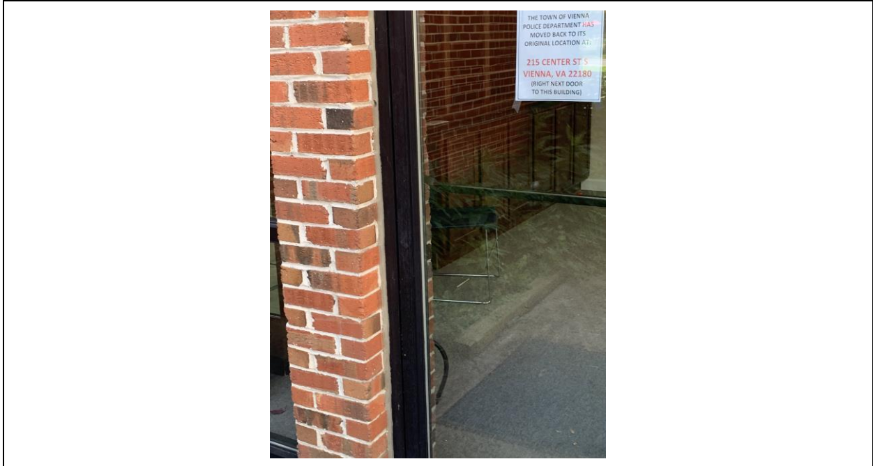
Homogeneous Material No. 31 – Non-ACM Brown exterior door caulk located on the front entrance door.
