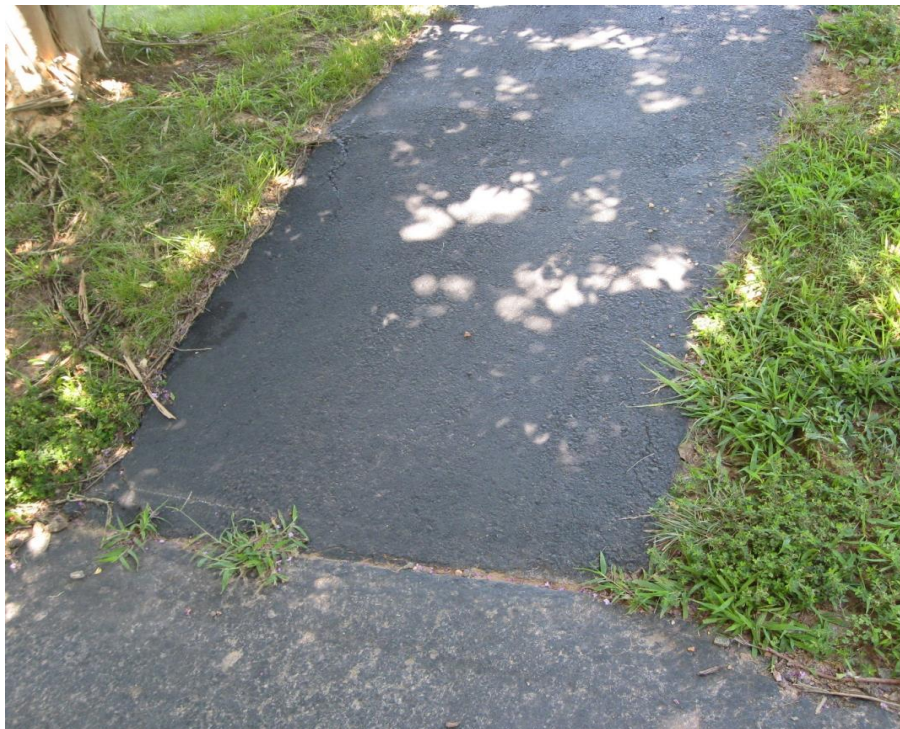
Continuing North. Issue with cross-slope. There may not be enough length of sidewalk to achieve desired slope.
