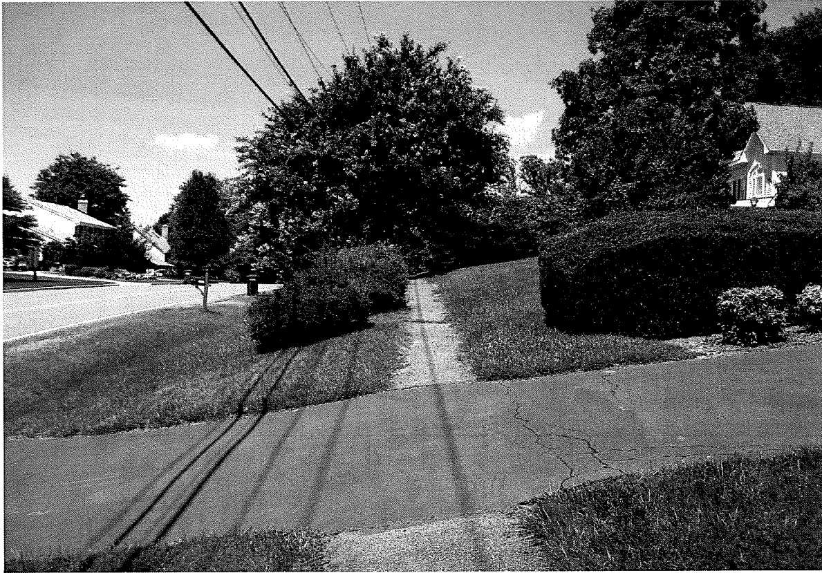
Uneven, sloping pathway along Creek Crossing Road. May present a cross-slope issue.
