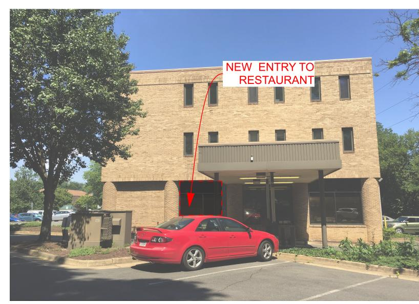
REAR ELEVATION WITH EXISTING AWNING TO REMAIN TO BE INFILLED AS NEW SCREENED PORCH EXISTING SITE PERSPECTIVE FROM MAPLE AVE
