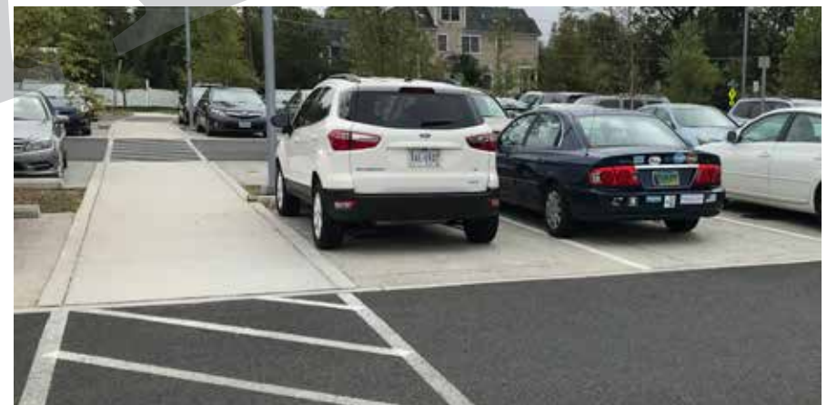
The parking lot at the Vienna Community Center was designed with porous concrete pavement under the parking spaces to allow stormwater runoff to infiltrate through the surface. An informational placard was added nearby to educate visitors on how the porous concrete works.
