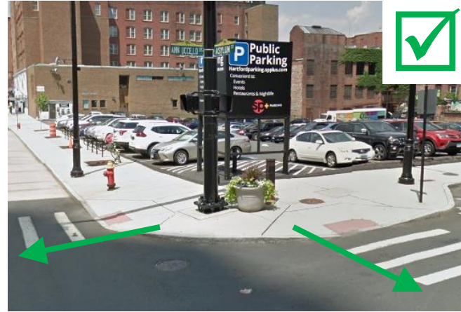
Example of a perpendicular curb ramp.
