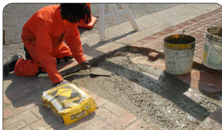
Installation of brick sidewalk along Church Street
