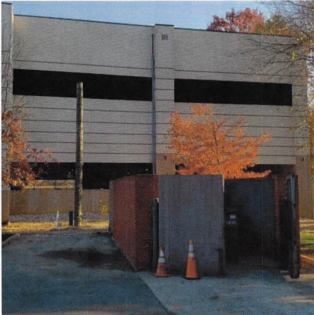
This is a rendering of a proposed awning. It is not meant to be an exact representation of the final product. Shop drawings and graphic layout will be supplied with exact measurements.
