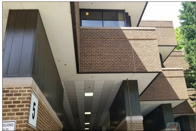
EXISTING VERTICAL METAL PANEL
