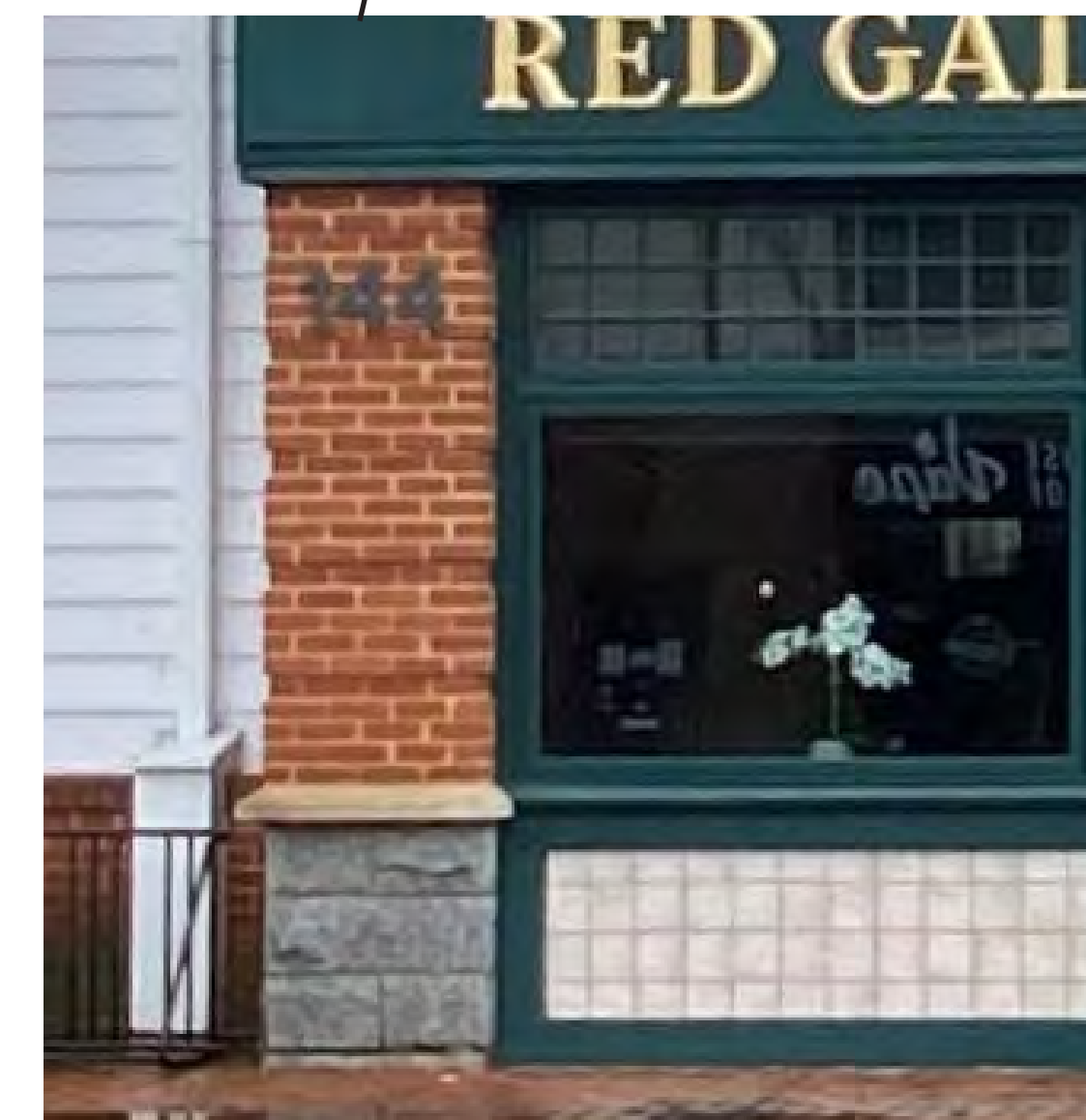
BRICK COLUMN ON STONE BASE
